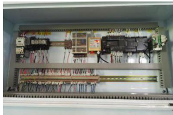
PLC centralized control
