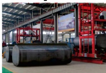
环缝自动焊 automatic welding of circumferential seams
