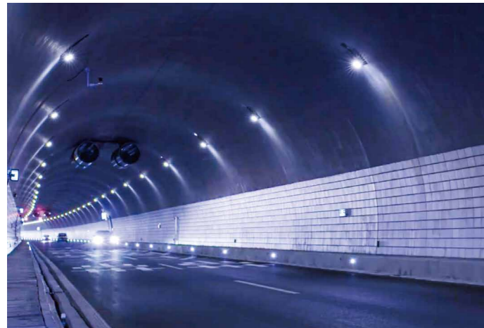
贵州黔西枫香河隧道项目 Guizhou Qianxi Fengxiang River tunnel project
