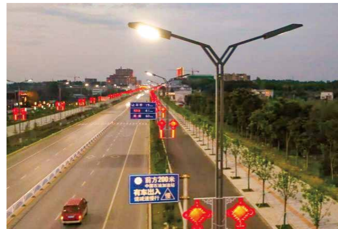
河南商丘永城永利路项目 Henan Shangqiu Yongcheng Yongli Road project
