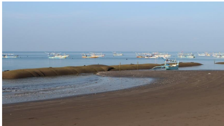
Figure 7. Shoreline condition after monitoring 7 January 2019
