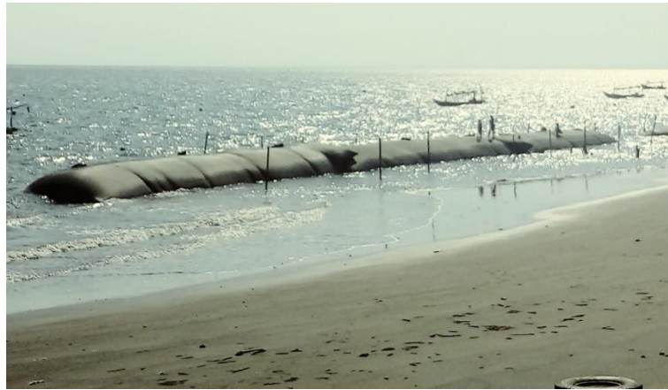
Figure 6. Shoreline condition after installation 7 October 2018
