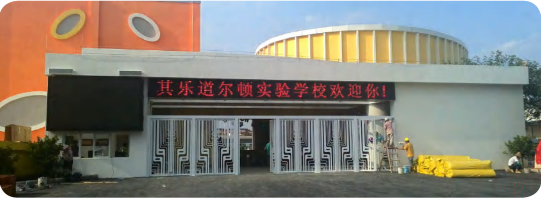
佛山道尔顿学校大楼 FOSHAN DALTON SCHOOL BUILDING
