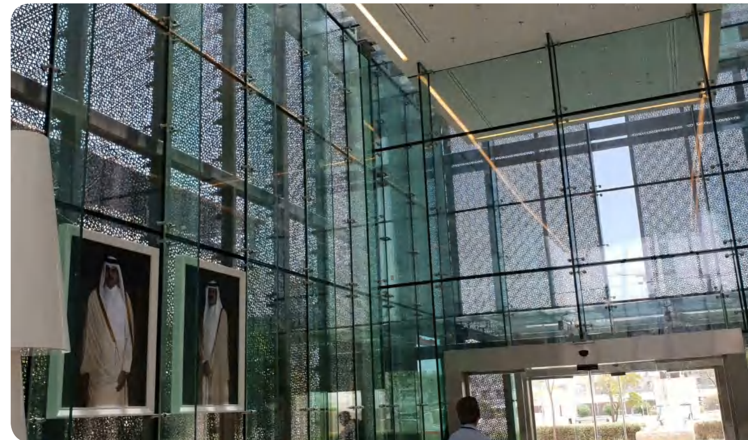
◎医院楼体外幕墙 External curtain wall of hospital building
