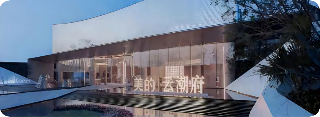
© 风铃幕墙—美的云潮府 WIND DRIVING CURTAIN WALL - MIDEA CLOUD TIDE MANSION
