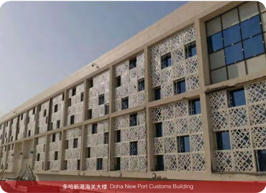
多哈新港海关大楼 DOHA NEW PORT CUSTOMS BUILDING
