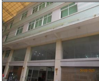
External photo(s) of the production unit(s) Office building.JPG
