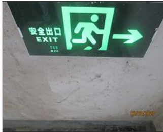
External photo(s) of the production unit(s) Evacuation sign.JPG
