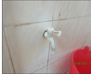
External photo(s) of the production unit(s) 7.22 Washing facility in toilet.JPG
