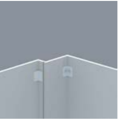
Glued and bolted at both angles at the back
