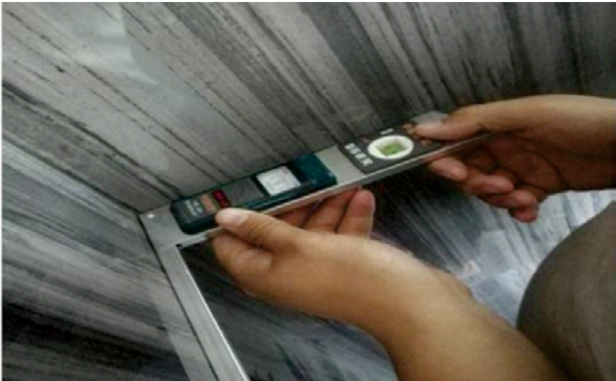
Inspect if the hidden corners can be 90 degrees
