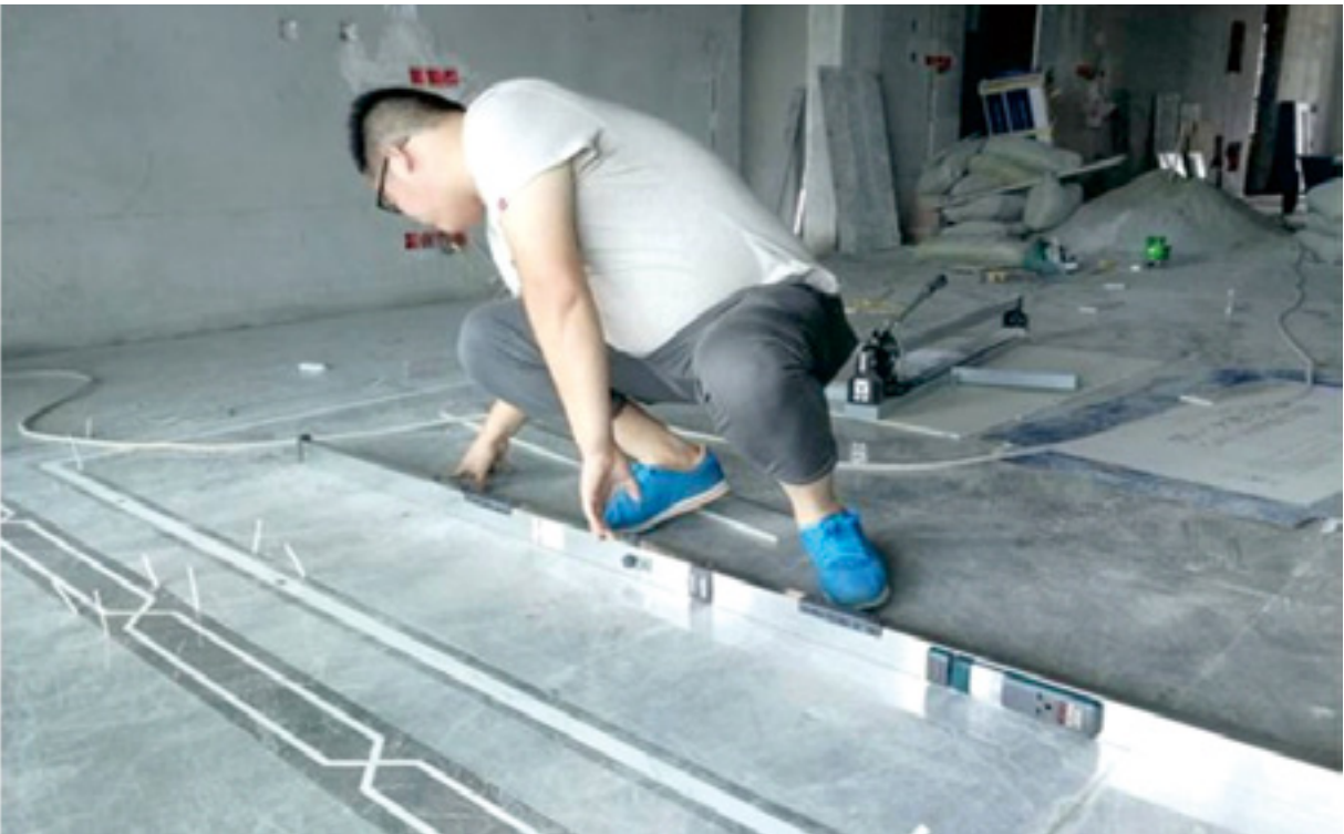
Inspection of floor flatness
