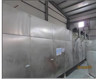
Photo of the inside of the main production hall Dryer.JPG
