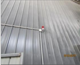
Photo of fire safety equipment Fire alarm.JPG
