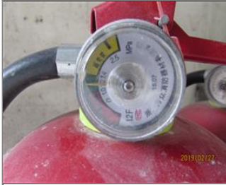
Photo of fire safety equipment Fire extinguishers with pressure.JPG
